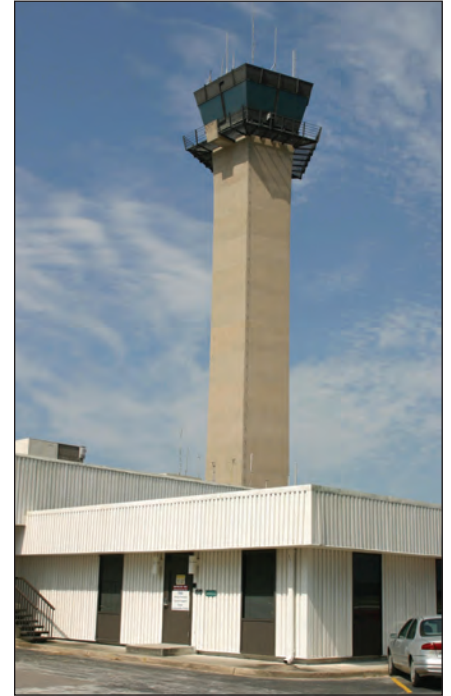
Airport Control Tower
